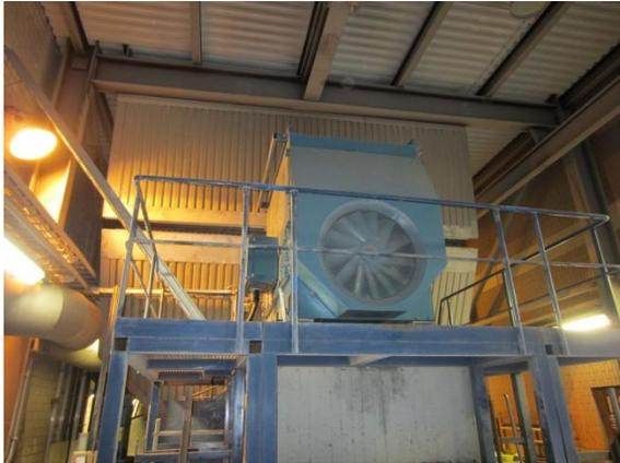
Figure 5. A picture of the inlet side of the axial fan.
